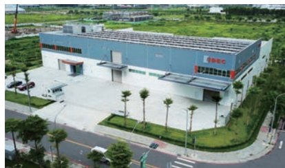
IDEC IZUMI TAIWAN CORPORATION of the IDEC Group has installed 1,200 solar power generation panels on the roof of its Ho Fa factory, constructed in September 2020.
