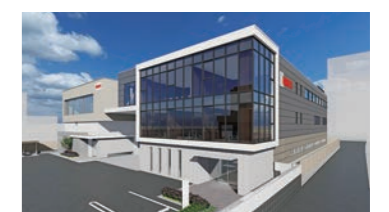
New head office (scheduled to be completed in March 2022)
